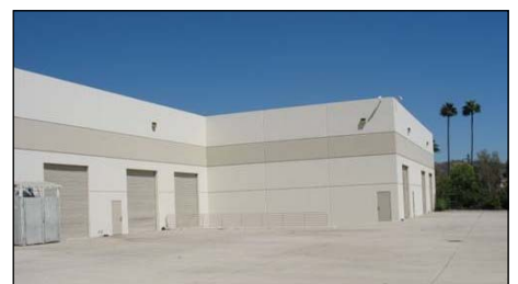
Loading and Storage Bay
