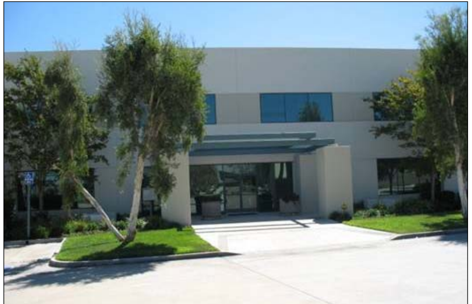
SEA CON ® Brantner & Associates, Inc., New Premises
