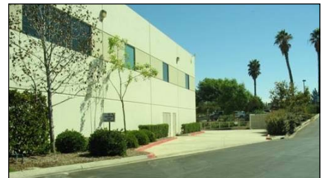
Side View of New Facility
